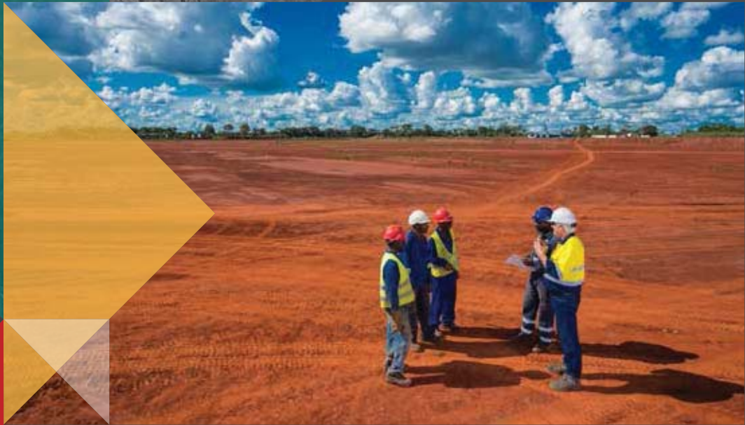
▲ Figure 1: Cleared processing plant site at Balama
