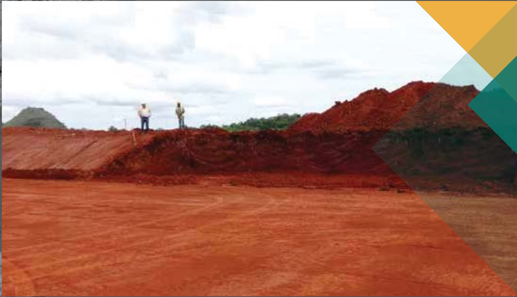
▲ Figure 3: First excavation for ore silo foundations
