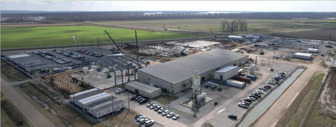
◀ Vidalia AAM facility
