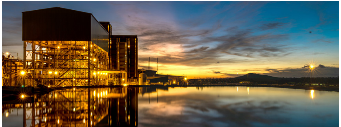
Balama processing plant
