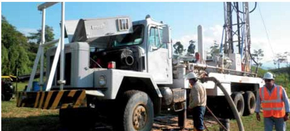
Drilling at Landazuri
