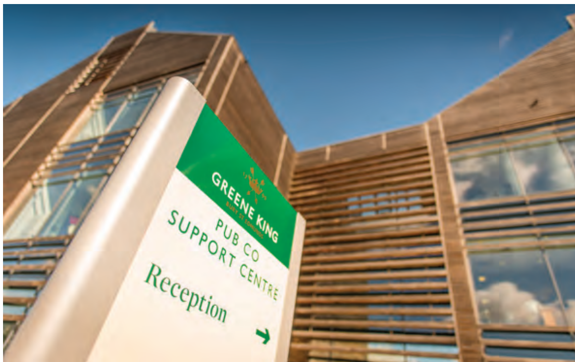
The new Pub Company support centre in Burton, Spirit's former headquarters.
