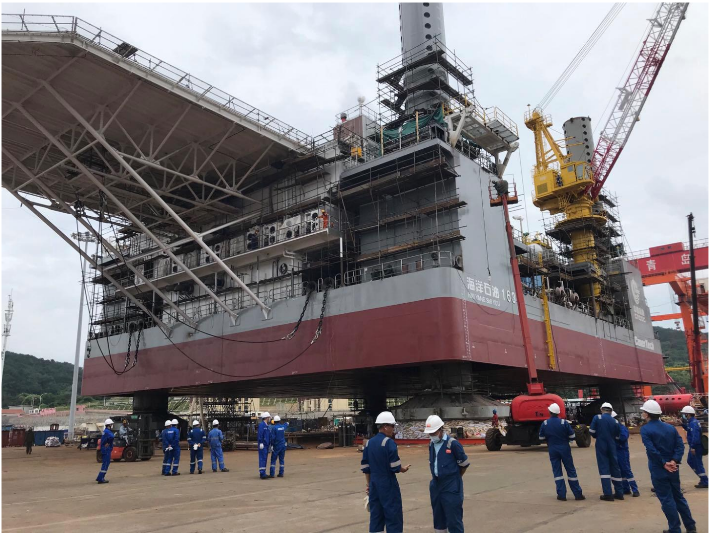
WZ12-8E Platform nearing completion in construction yard
