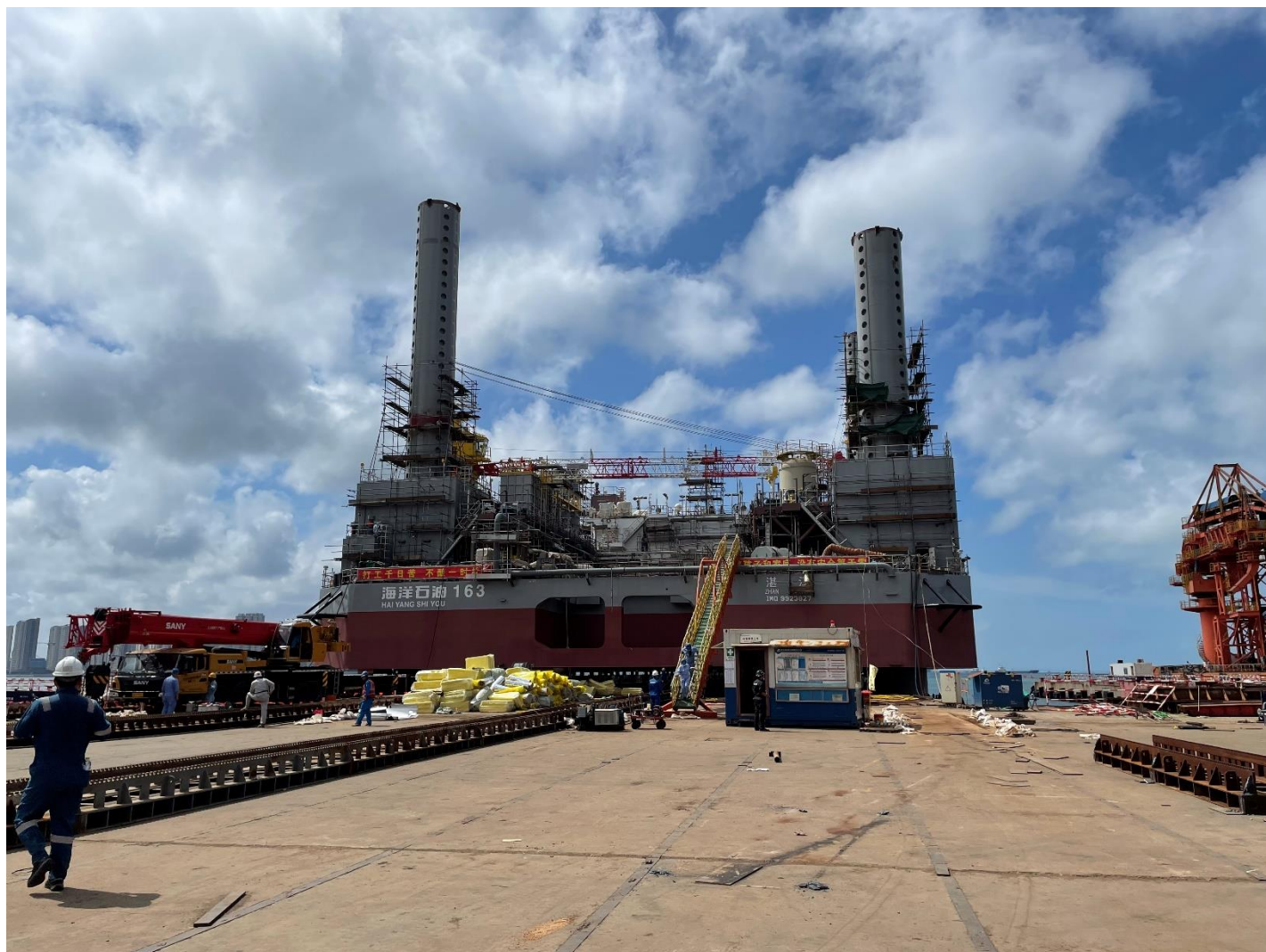
WZ12-8E Platform under construction in construction yard
