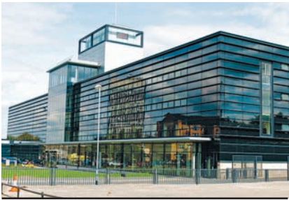
THE LEICESTER MERCURY BUILDING HAS RECENTLY BEEN RENOVATED.
