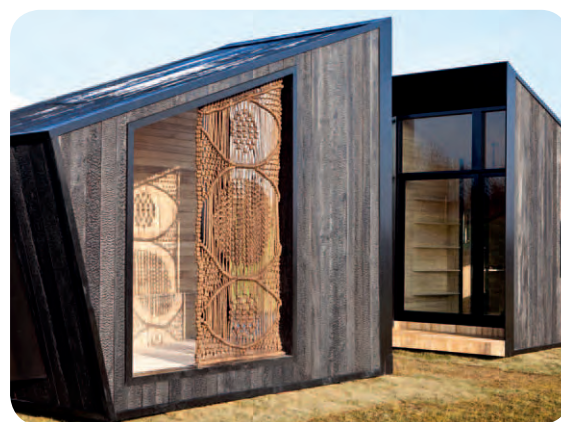
We sponsored these amazing Observatory style artist's studios supplying home grown and imported Larch which was charred to clad the exterior as well as Accoya, Medite Tricoya Extreme and Smartply which was used on the interiors.
