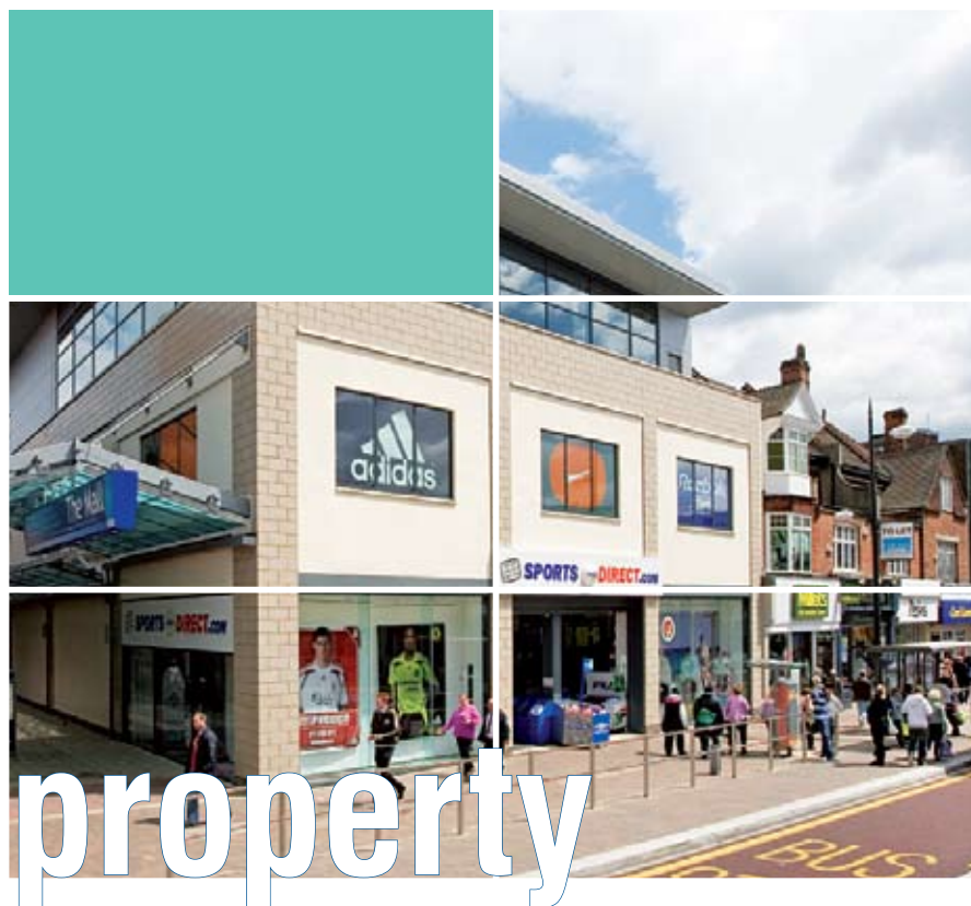
THE MALL RETAIL AND OFFICE DEVELOPMENT IN BROMLEY WAS SUBSTANTIALLY COMPLETED IN THE YEAR
