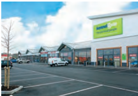
▲ Sandlands Court, Mansfield – the mixed-use district centre scheme completed and fully occupied during the year.
