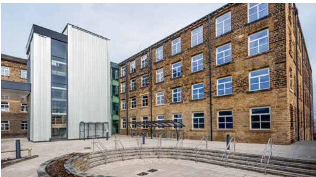
Recently completed exterior of Acre Mills in Huddersfield. The interior works commenced in 2014
