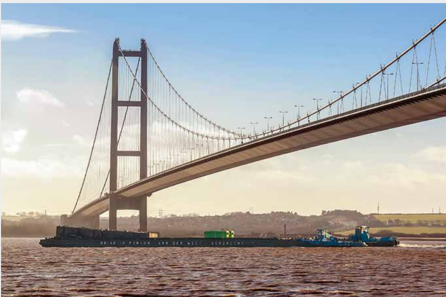
Two 315 tonne parts of the press being transported to Lincoln via the River Humber
