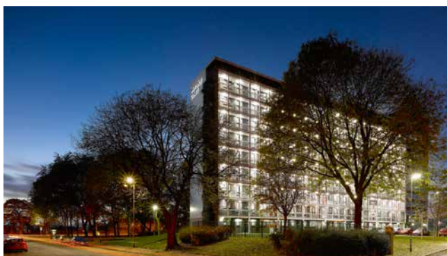
A night shot of the refurbished Worsley Court Manchester tower block for Eastlands Homes
