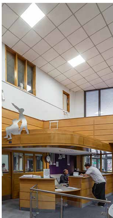
Recently completed refurbishment of eleven floors of office space at Moorfoot for Sheffield City Council
