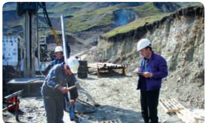
DISPENSING CORE FROM THE CORE BARREL
