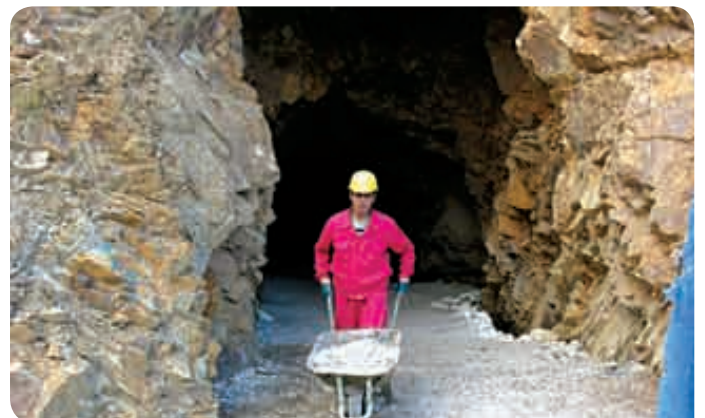
ADIT CLEANING AT ORDUBAD
