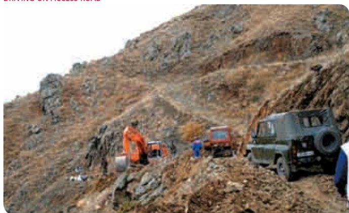
DRIVING ON ACCESS ROAD
