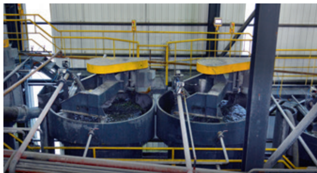
Two of the smaller flotation cells in production. On top of the two cells can be seen the 'froth' which is dewatered to form the concentrate.
