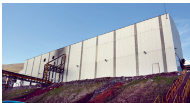
Outside view of the flotation plant.
