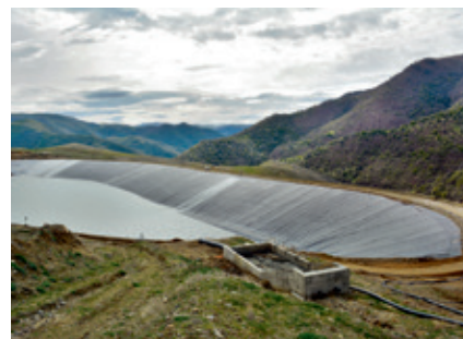
The raised wall of the tailings dam now fully completed.
