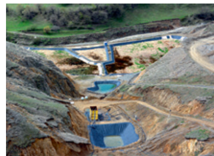
Completed reed bed biological system immediately downstream of tailing dam.
