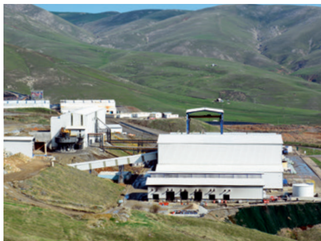
View of the agitation leaching plant and completed flotation plant.
