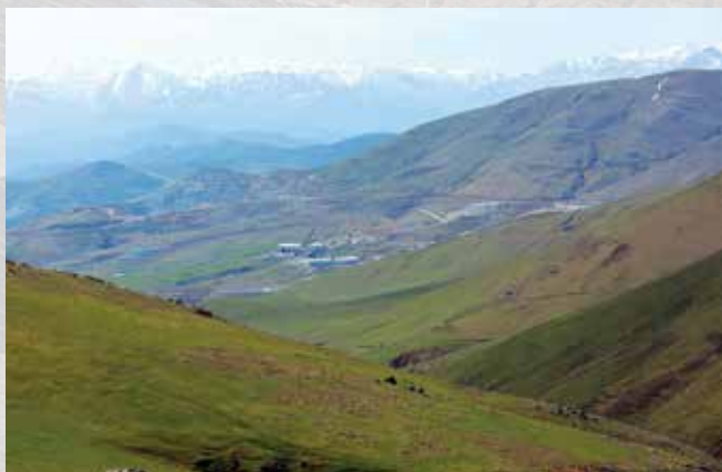
View of the processing facilities and the main open pit from the Ugur gold deposit.
