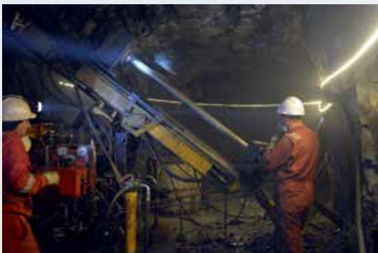
Core drilling taking place in the Gadir mine.
