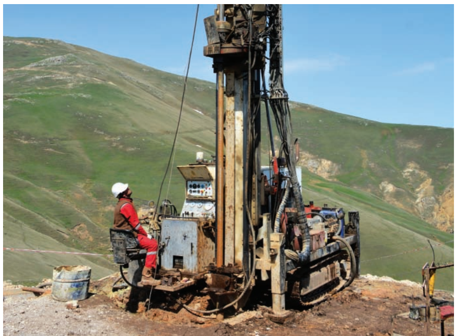
Core drilling at Ugur.
