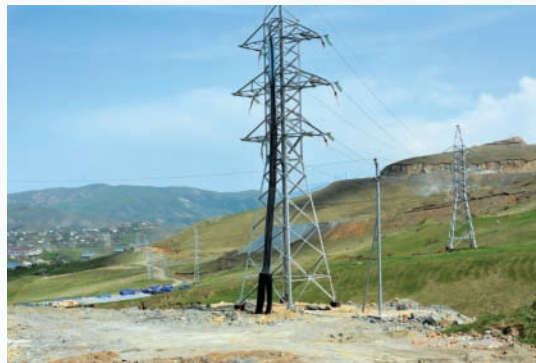
Seven kilometres of 35 kilovolt overhead power cable were constructed.
