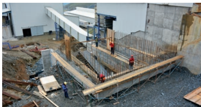
Construction of the foundations for the new jaw crusher.
