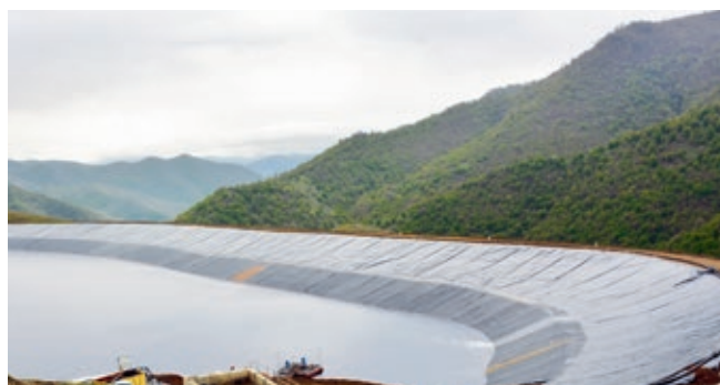
Tailings dam showing the wall raised by six metres.
