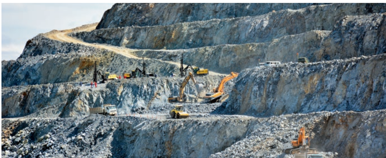
Push-back of the back wall as part of the development of the main open pit.
