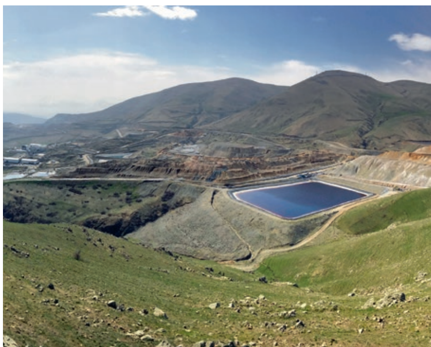
Panoramic view of the Gedabek site.
