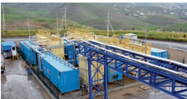
New water treatment plant.
