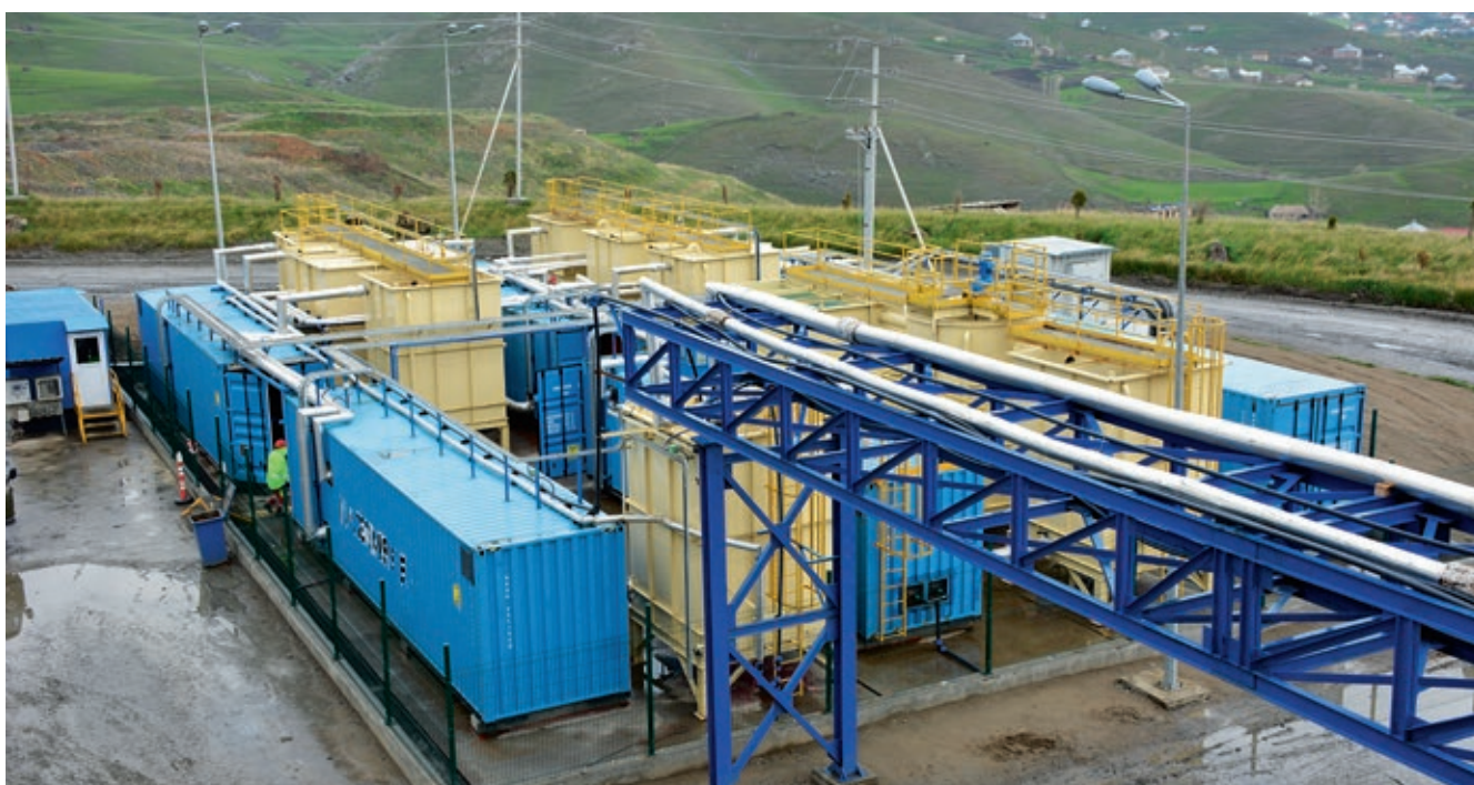
New water treatment plant.
