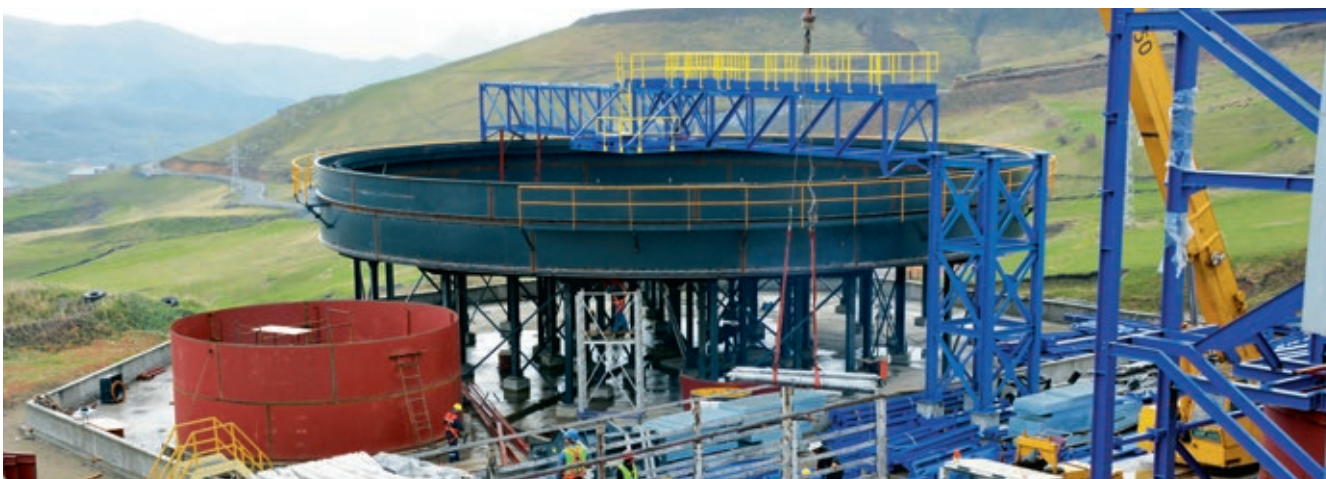
Additional thickener being constructed for the new second crusher line.
