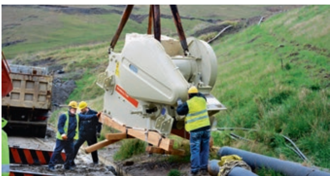
Delivery of the new jaw crusher.
