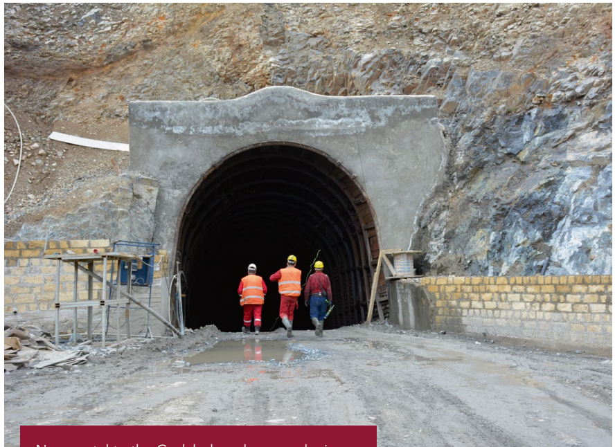
New portal to the Gedabek underground mine
