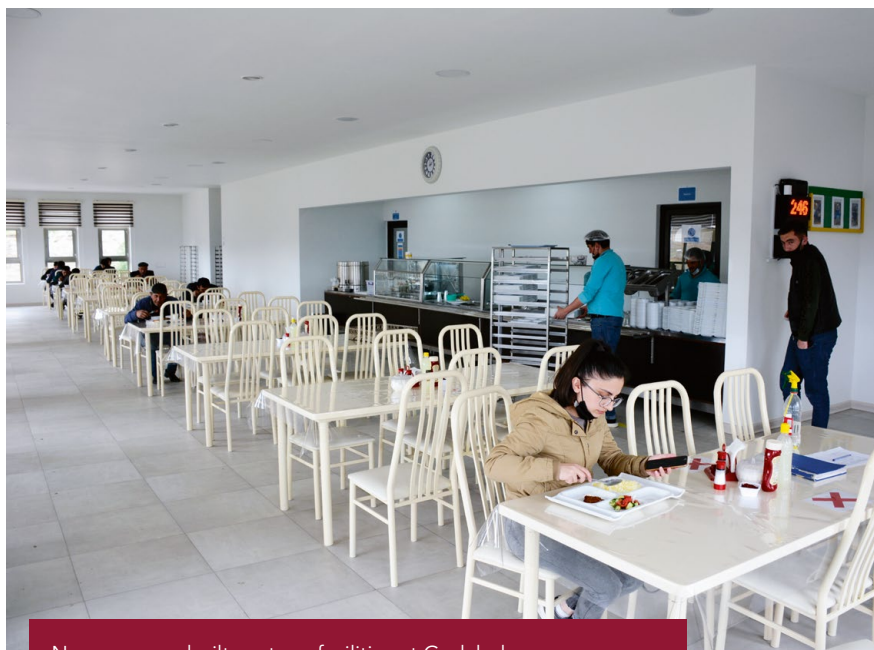
New purpose-built canteen facilities at Gedabek
