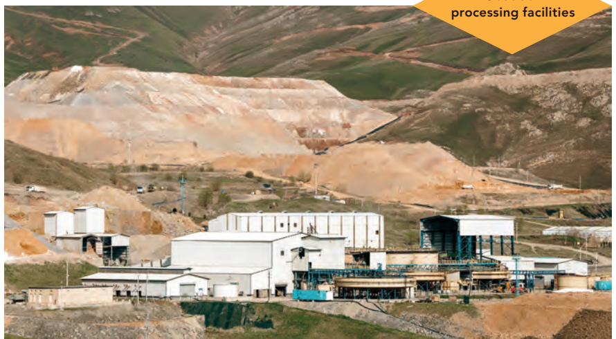
Gedabek processing facilities
