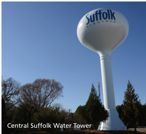
Hillpoint – Suffolk 3100 Godwin Boulevard
