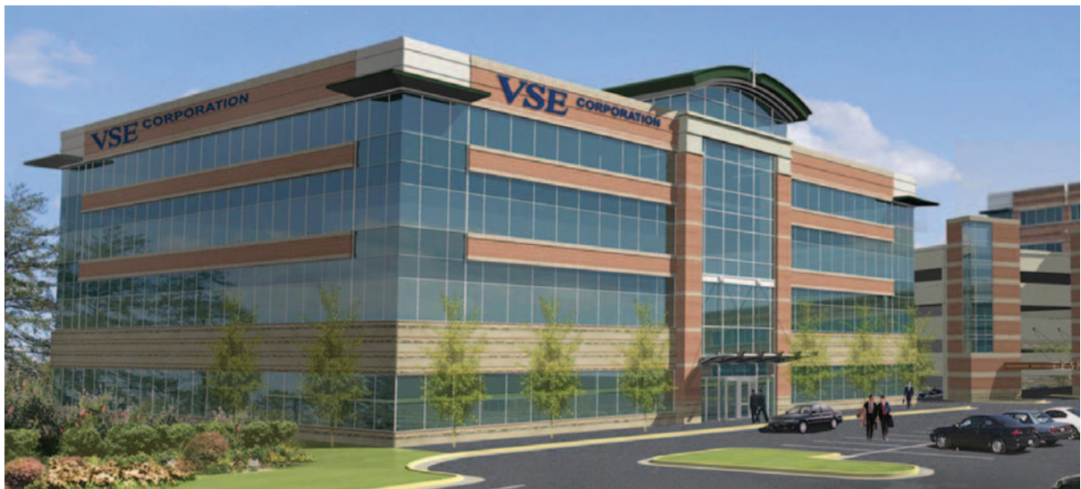
Artist rendition of new VSE Headquarters in Springfield, Virginia set to open in Spring 2012.
