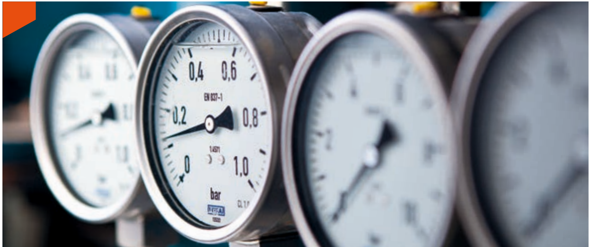
Pressure gauges monitor steam turbine auxiliaries.
