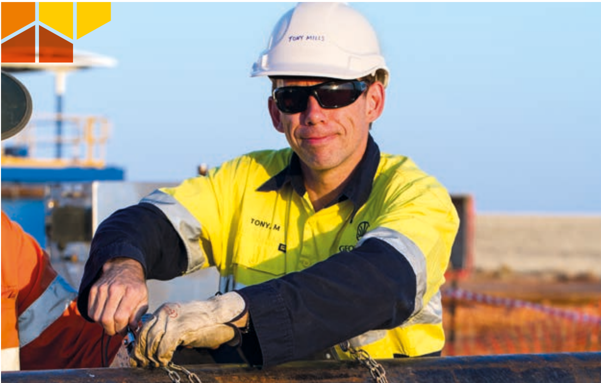
Inspecting surface equipment during trial.
