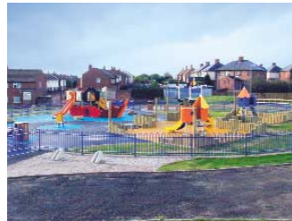
Creating a community Doctor's surgery and playground site at Widdrington – part of a local community investment project in association with East Northumberland Regeneration Initiative.
