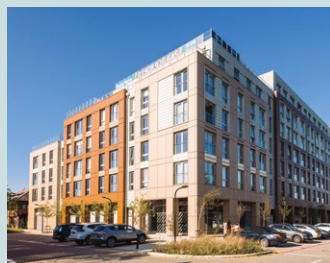
Solstice Apartments, Milton Keynes – launched in 2020 and offering 139 new rental homes in the heart of Milton Keynes. Residents enjoy a range of amenities, including several outdoor terraces and courtyards, excellent transport links, as well as great shopping and restaurants right on their doorstep.
