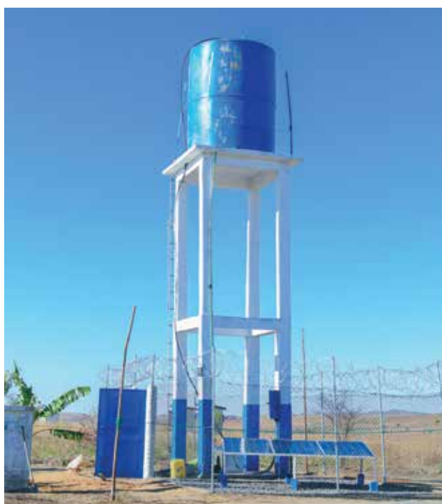
Water tower, water storage tank and solar panels for the water pump.
