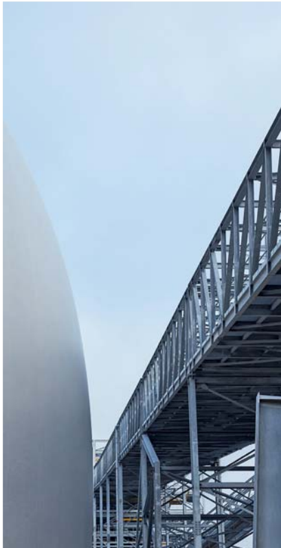
The new biomass facilities at Drax Power Station are now supporting two converted biomass units.
