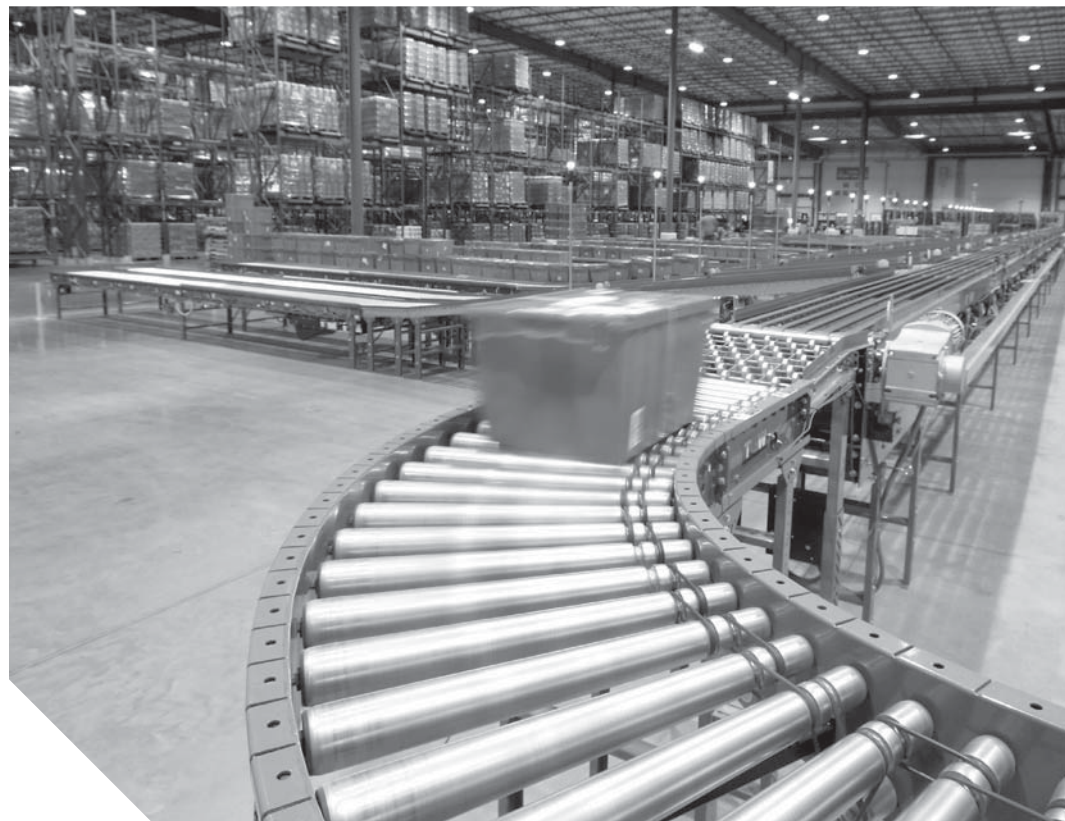
Distribution Center Terre Haute, Indiana
