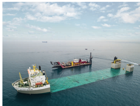
Dredge Ohio preparing for return to the U.S. Bahrain
