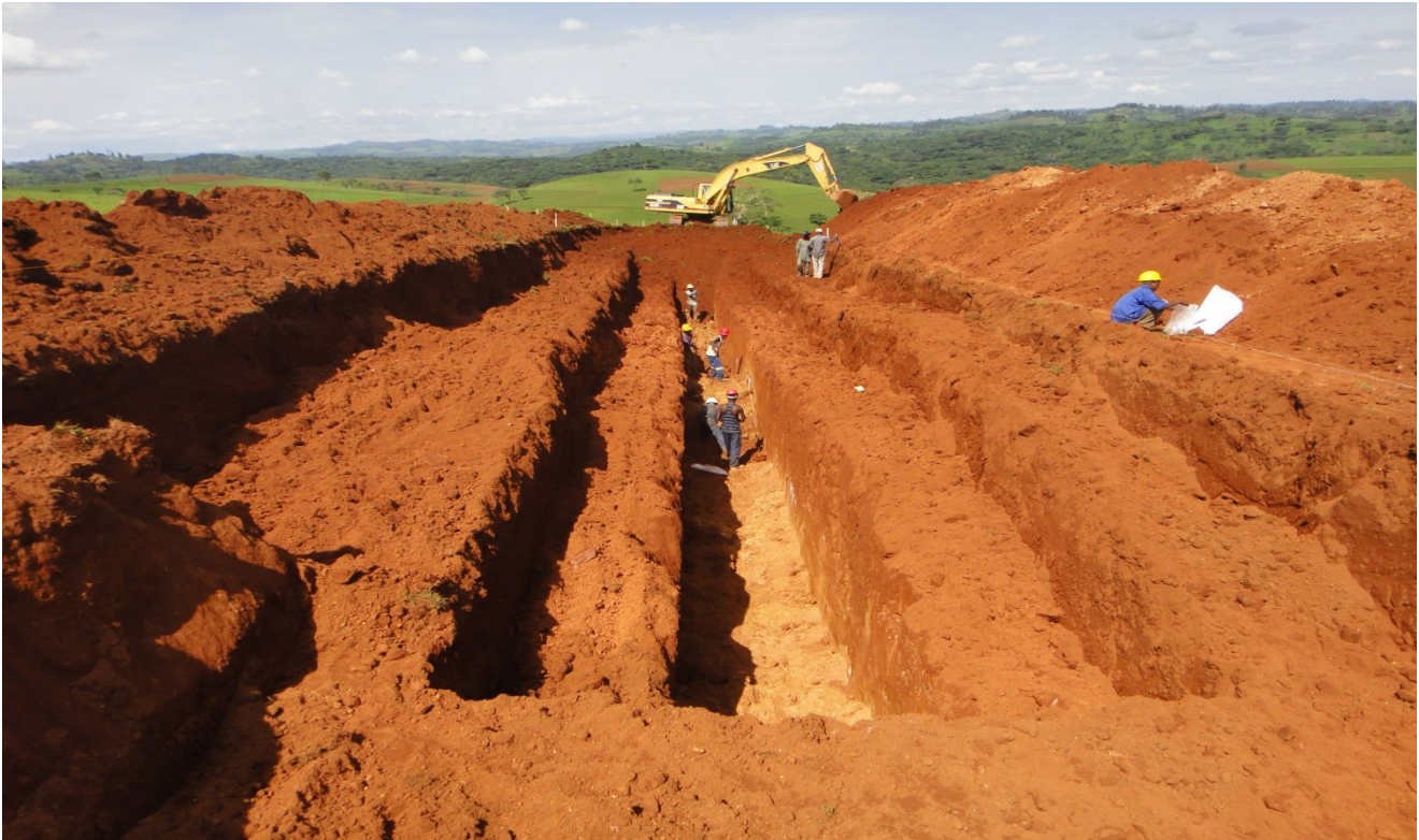
Trenching at Tulu Kapi
