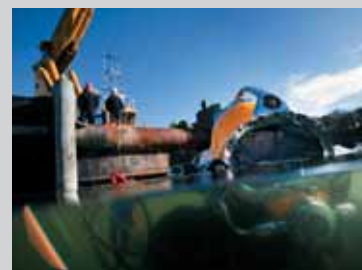
Divers inspecting pontoons at our marine services contract in Davenport, UK.
