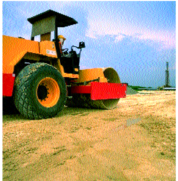
A worker maintains an oil field road in Indonesia. In early 2001, Devon signed a groundbreaking agreement to supply Indonesian natural gas to Singapore.
