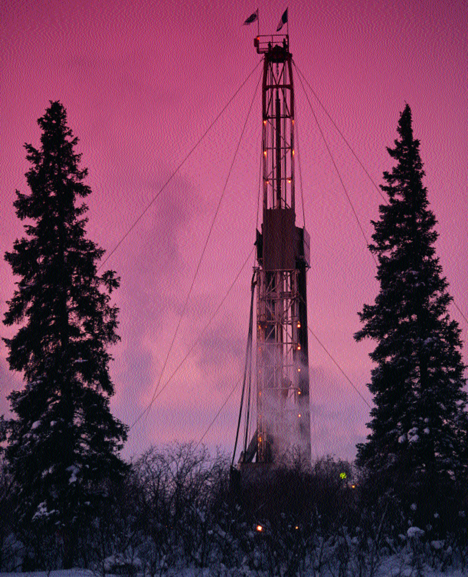
Devon drills this exploratory well in Canada's Mackenzie Delta. Drilling is limited to the winter months when the ground is frozen and can accommodate heavy equipment.
