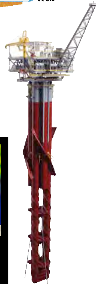
▲ A SCALE MODEL of the Red Hawk cell spar provides a view of the completed facility. Each of its six mooring cables will extend more than a mile to anchor the massive floating structure to the sea floor.
