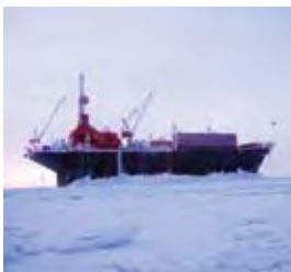
A steel drilling caisson was used to drill Devon's Paktoa well in the Beaufort Sea in far northern Canada. Devon is the largest exploratory land holder in the Mackenzie Delta and Beaufort Sea areas.
