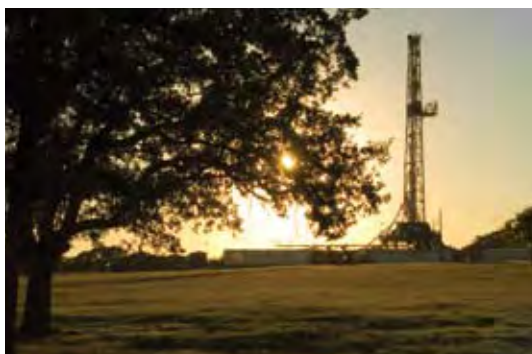
This rig is drilling in the Barnett Shale near Cleburne, Texas. Devon drilled its 2,000th Barnett Shale well in 2005.
