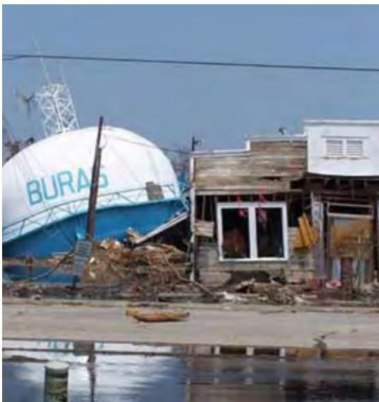
The 2005 Gulf of Mexico hurricanes did extensive damage to coastal communities such as Buras, Louisiana. Devon employees responded generously with donations of time and money.
