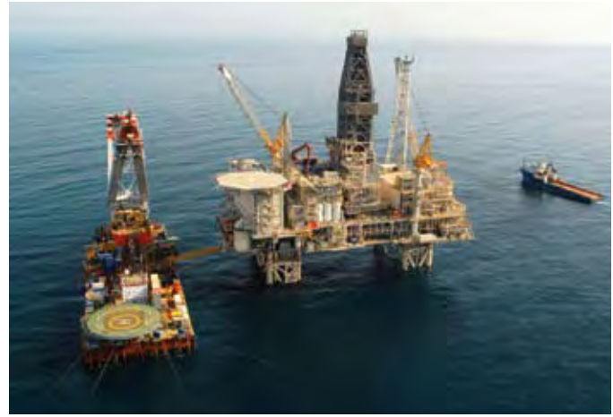
Drilling operations on the ACG field, offshore Azerbaijan, have increased field-wide production to more than 700,000 barrels of oil per day. Devon's share of production is expected to average more than 30,000 barrels per day in 2007.
