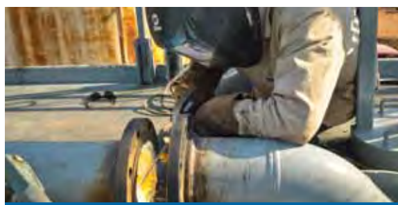
Welding at Hastings Field
