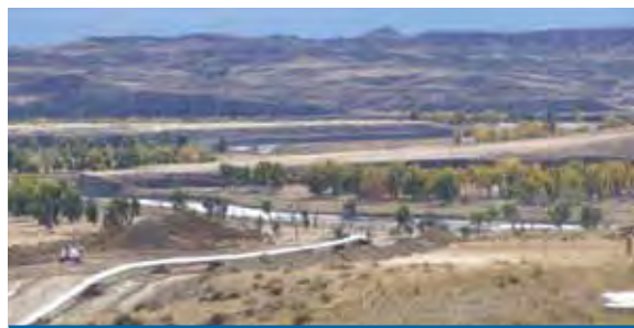
Greencore Pipeline construction
