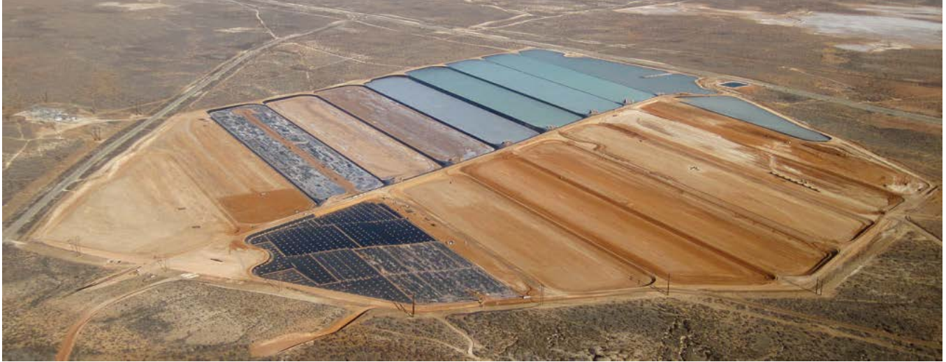
Aerial view of HB solar evaporation ponds.
