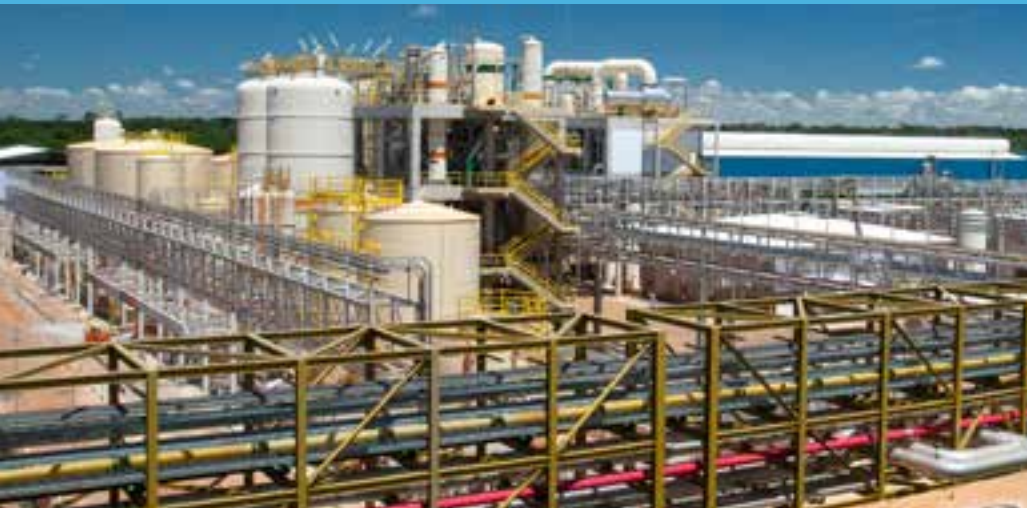
Our Chemical Island sites are integrated with pulp mills and primarily run on renewable excess energy.
