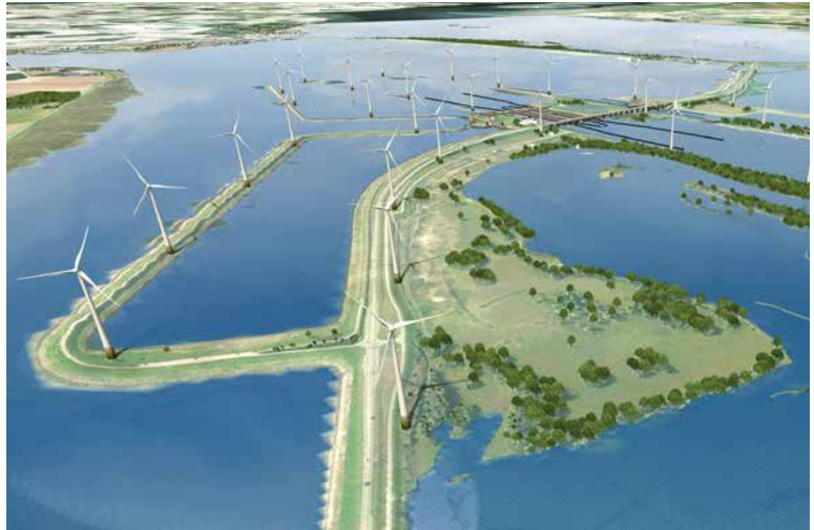
In 2016, a consortium of four companies in the Netherlands – led by AkzoNobel – agreed to source power from the Krammer wind park once it becomes operational in 2019. The partners (including Google, Philips and DSM) will purchase a total of 350 million kWh a year, equivalent to the total annual consumption of 100,000 Dutch households.
