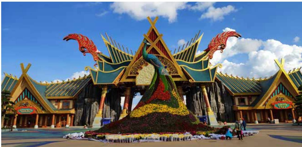
The first theme park in South West China opened in 2018 – and our Dulux Pro paint brand was used to coat around 180,000m 2 of attractions and facilities in 80 different colors. Known as Yunnan Happy World, the park is located in Kunming, Yunnan province.
