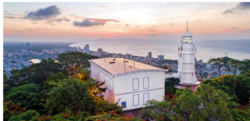
One of Southeast Asia's oldest lighthouses is being protected by our Dulux Weathershield exterior paint. Vung Tau lighthouse, located on the top of Nho mountain in Vung Tau province, Vietnam, was built by the French in 1862. The project to repaint the historic structure was launched as part of Dulux's Lighthouse Protection Campaign.
