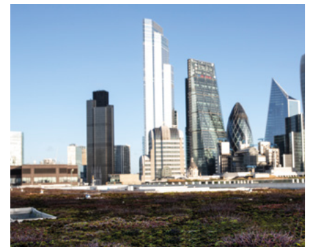
Riverbank House Green Roof
