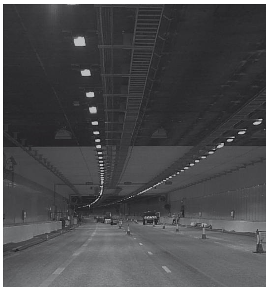
Hatfield tunnel on A1(M).
