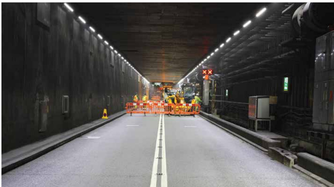
Heathrow Main Tunnel, Hounslow
