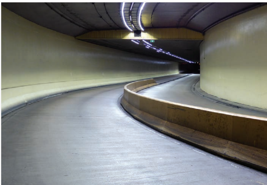
Pictured: Ivory Street Tunnel, Australia
