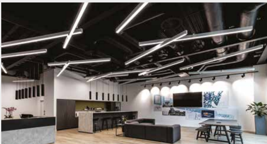
SmartScan installation at BuroHappold offices in Leeds
