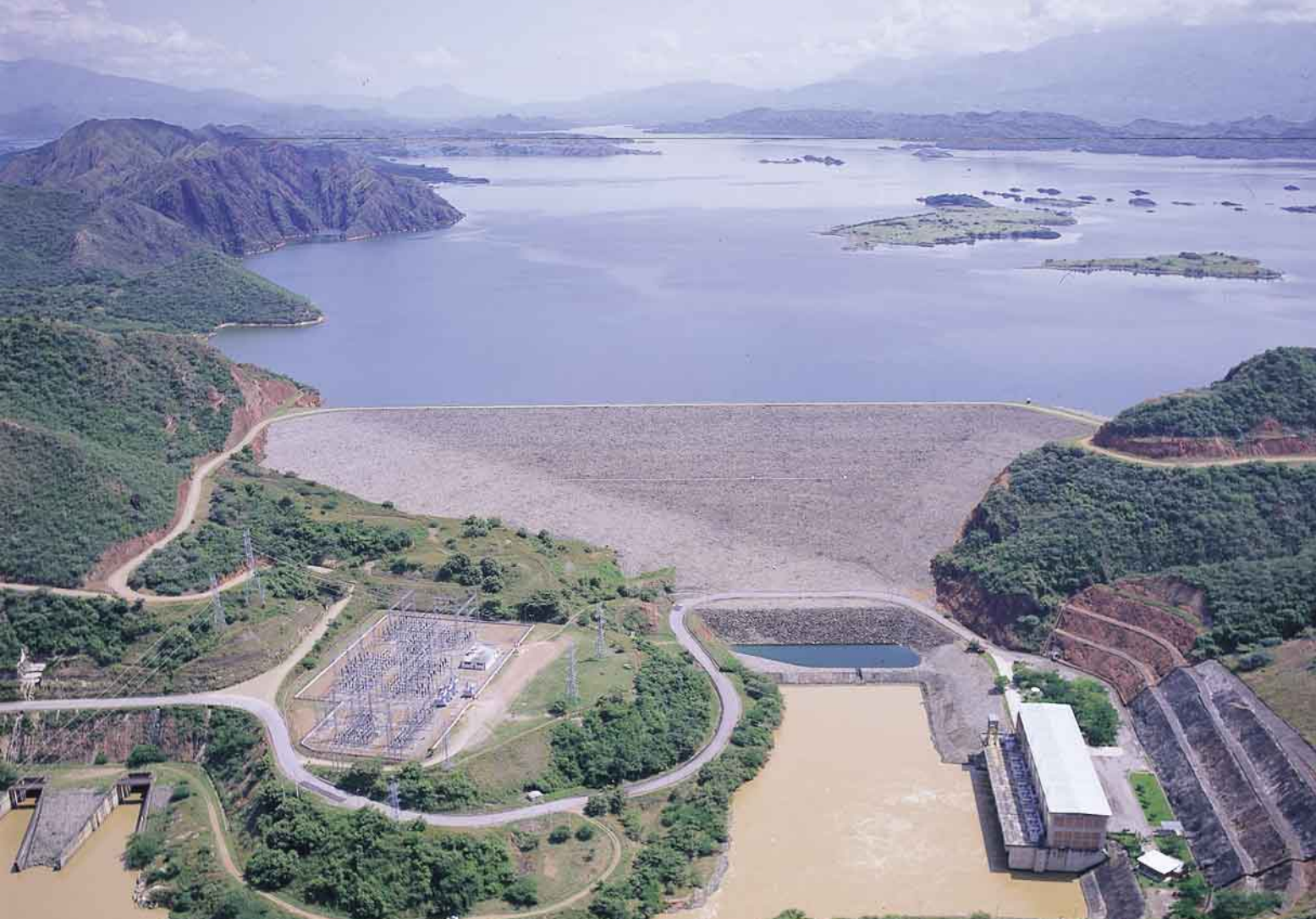
Betania Hydroelectric Power Plant, Colombia
