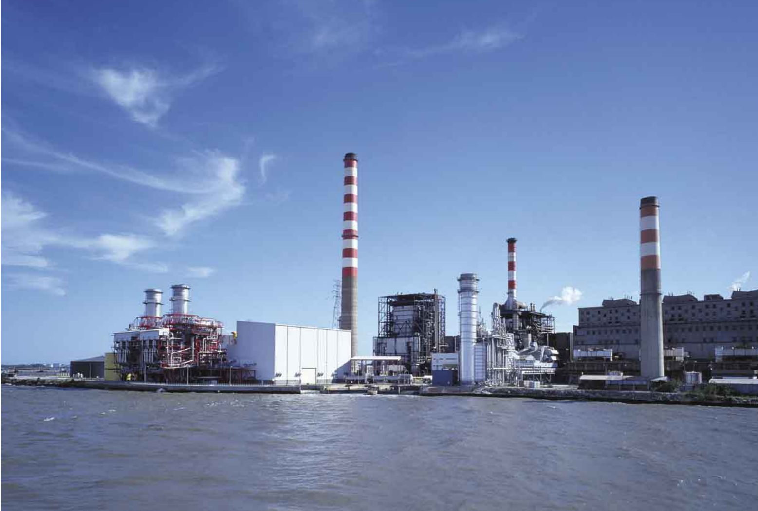
Costanera Power Plant, Argentina
