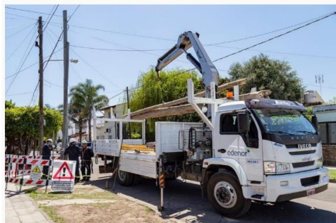
Replacement of LV pole
