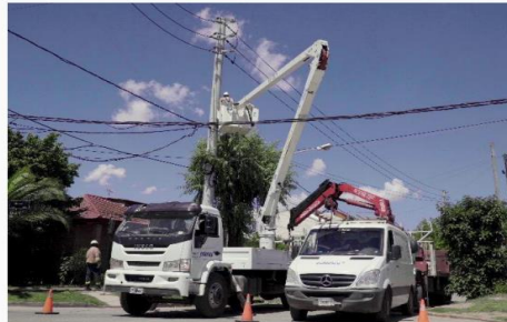
Laying of MV overhead line
