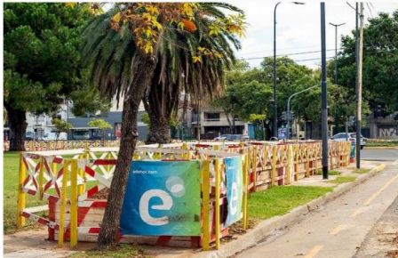
Laying of MV underground cable
