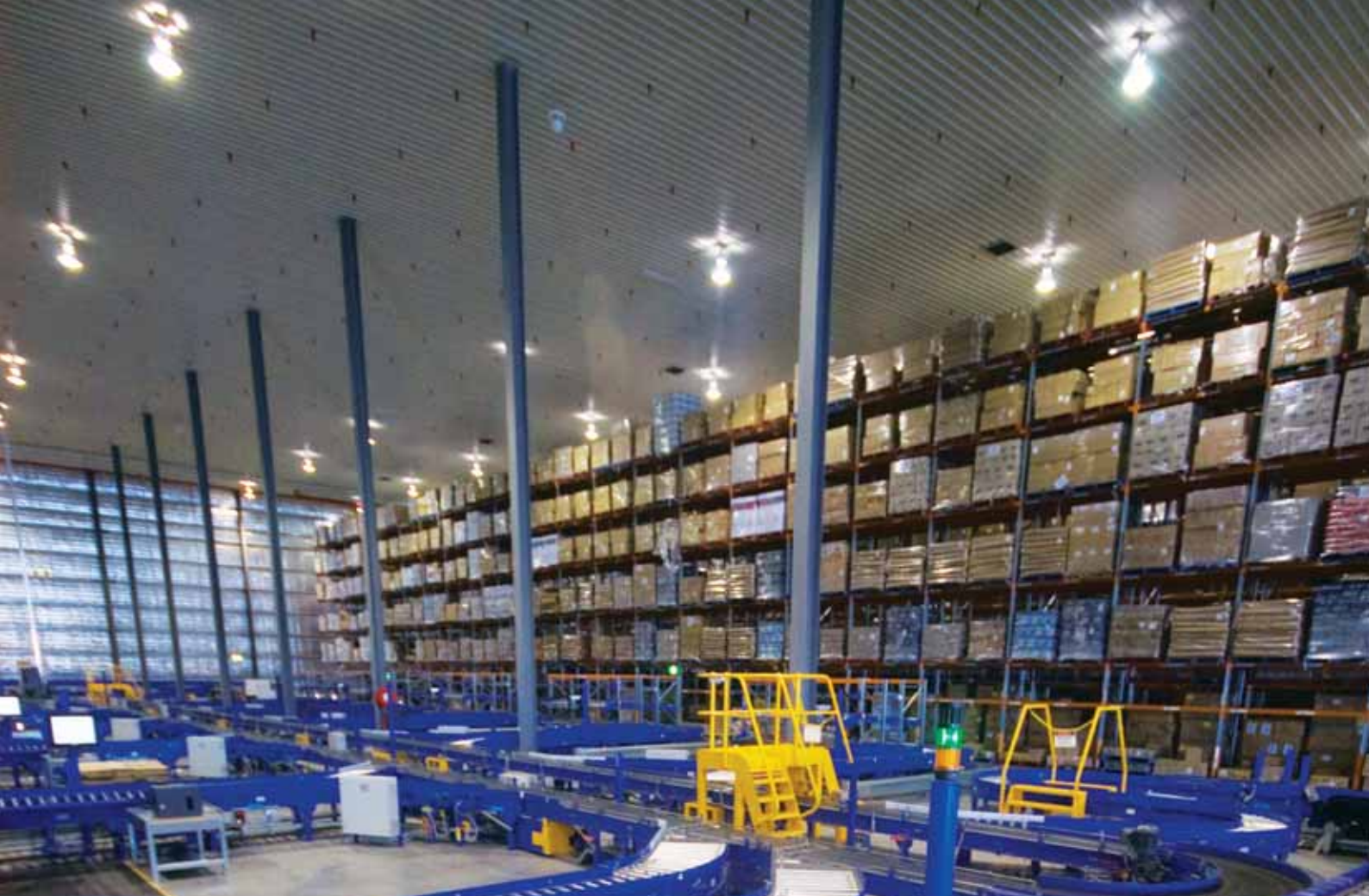
Image: The new 'mini loader' installed in the Laverton, Victoria warehouse.
