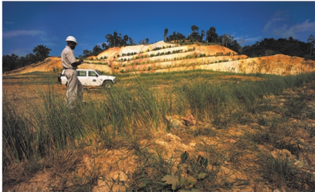
Early stages of waste dump stabilization immediately following the completion of mining.
