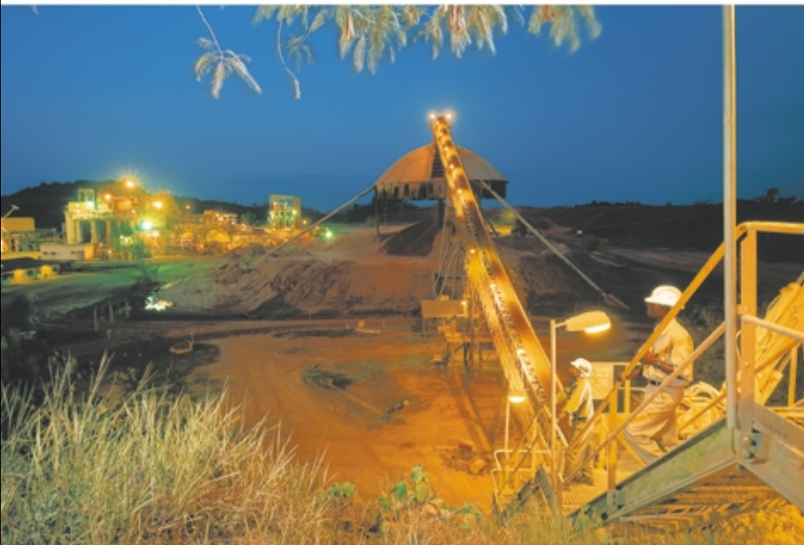
Bogoso processing plant and crushed ore stockpile.
