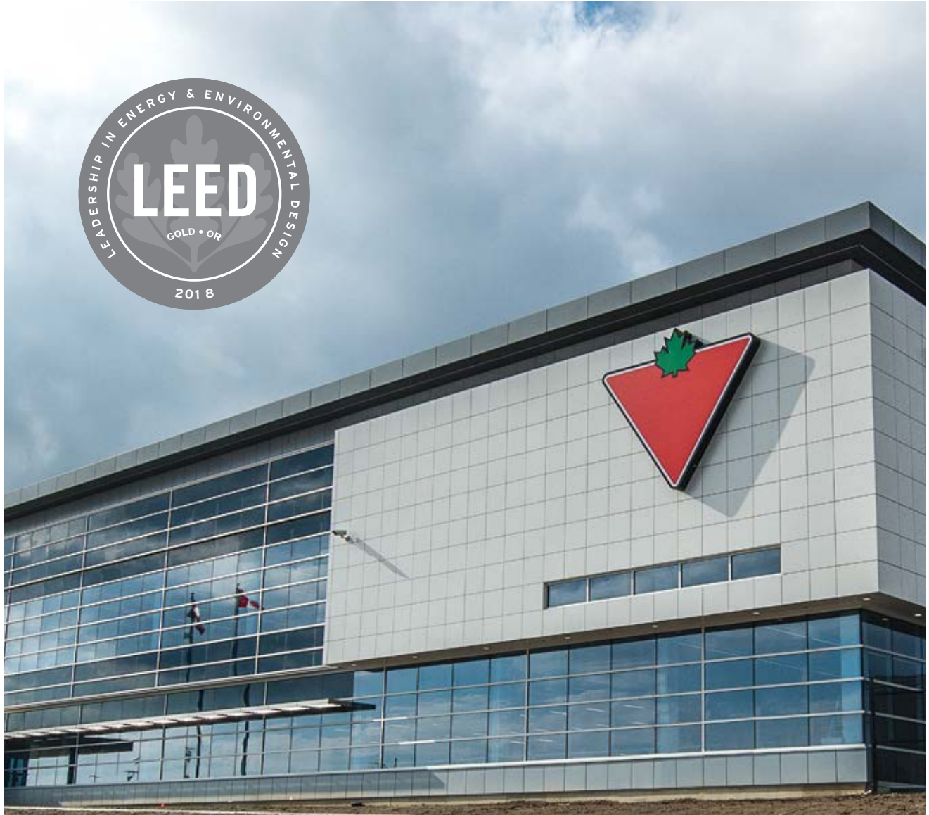
The Canadian Tire Bolton Distribution Centre in Caledon, Ontario was awarded LEED Gold certification for exceptional sustainability efforts.
