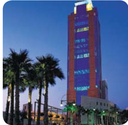
PORTOMASO TOWER, ST JULIANS, MALTA
