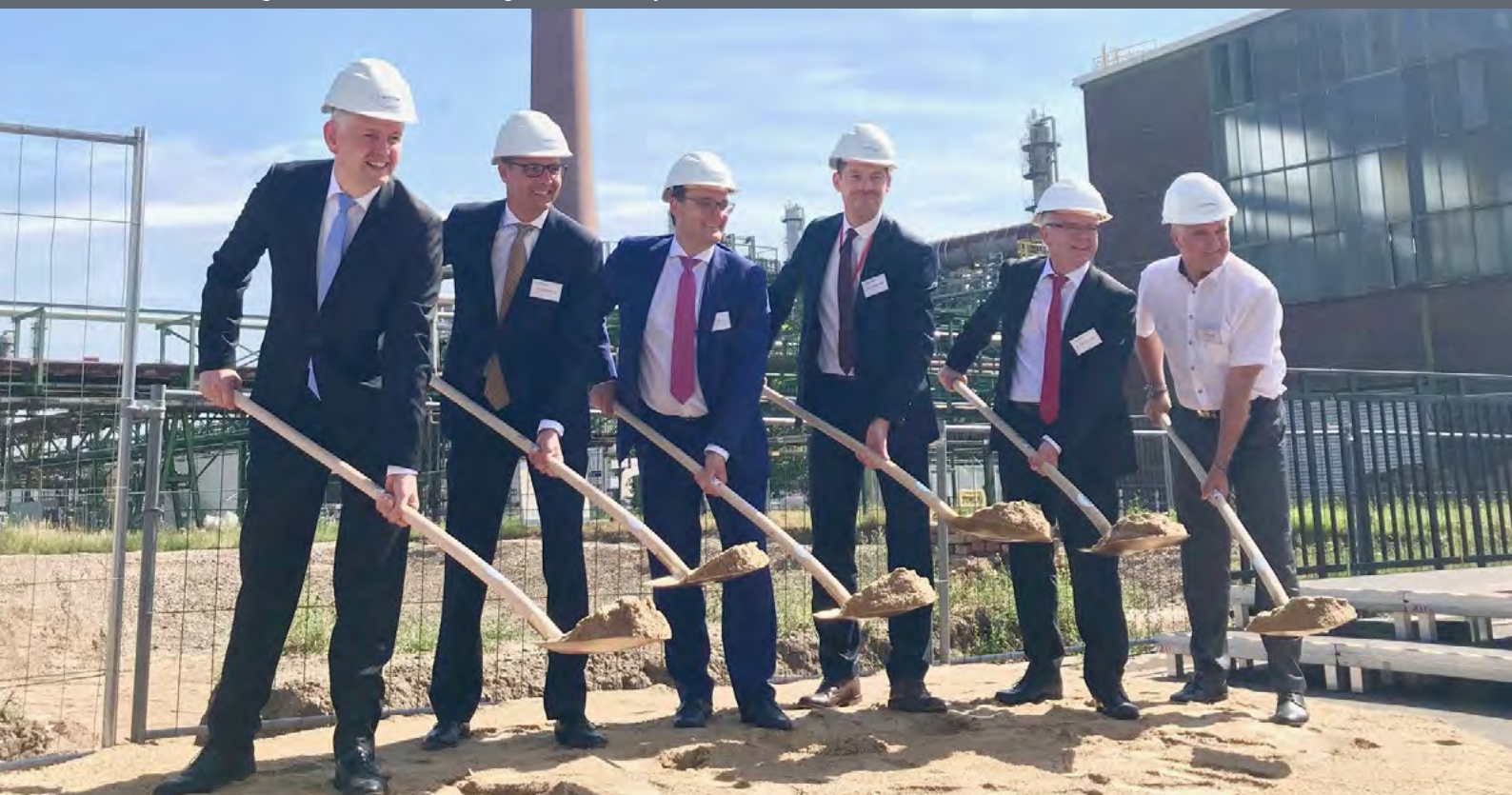
Ground breaking of REFHYNE the worlds largest PEM Electrolyser
